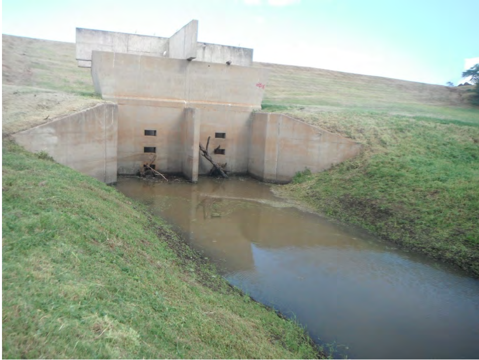
Figure 3- 7 Open ports at the riser structure, Honokōwai Dam (2017)
