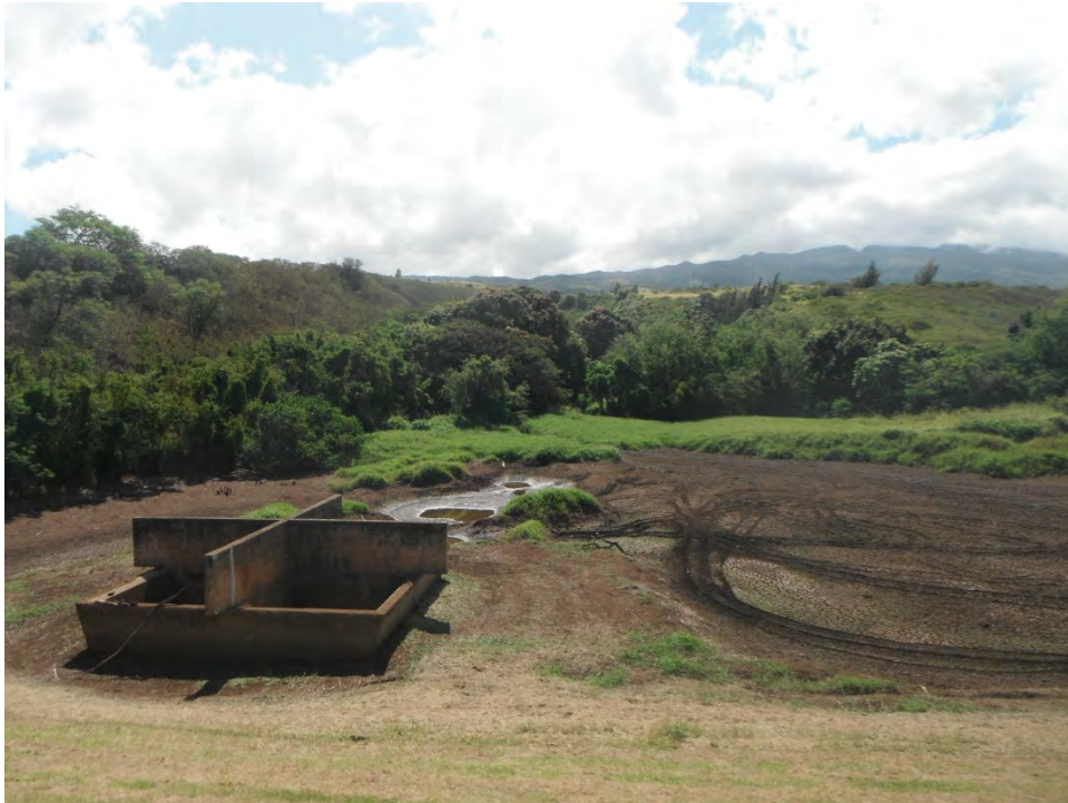
Figure 3- 8 Riser structure and saturated conditions, Kahana Dam (2017)
