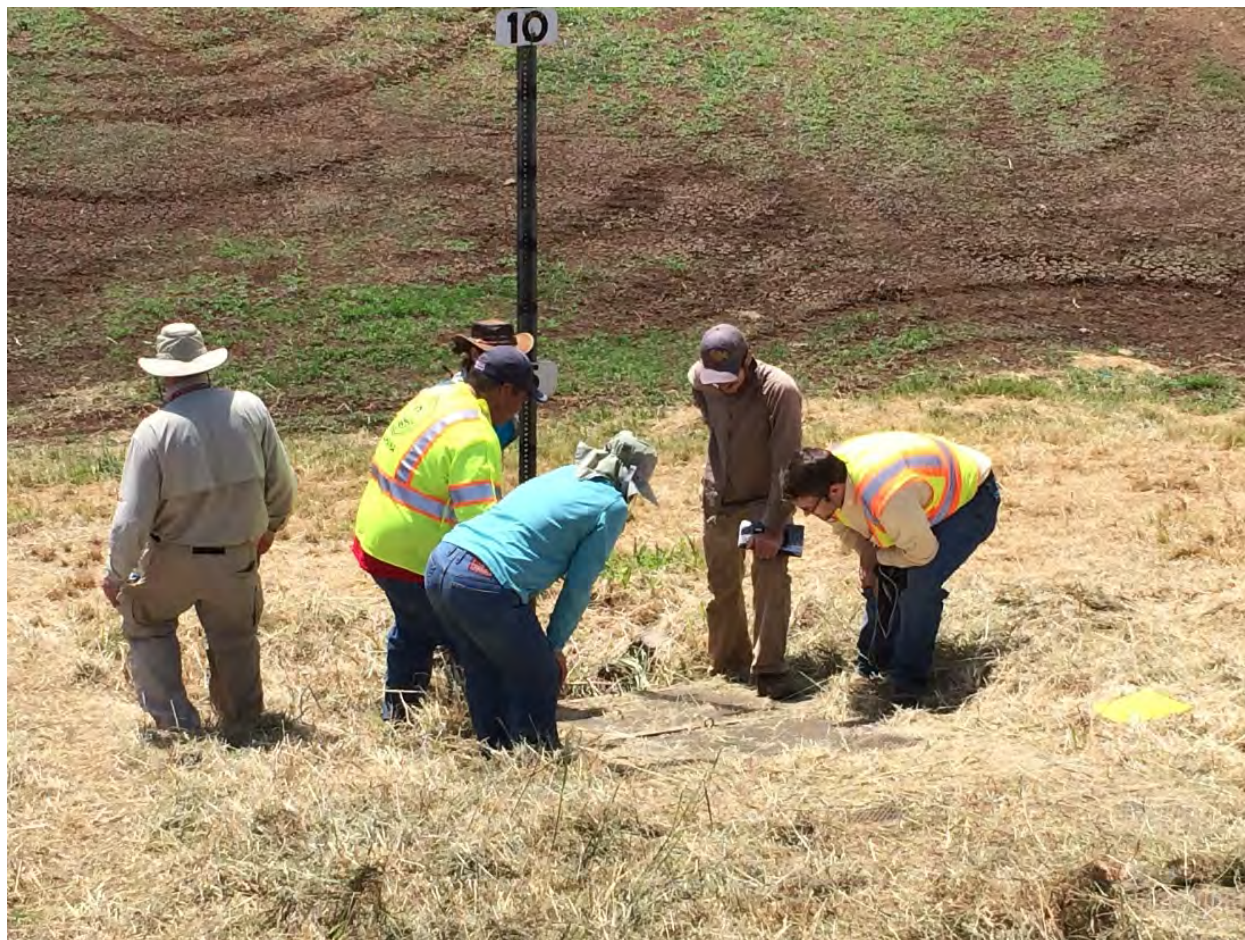
Figure 3- 10 Outlet Modification at Napili 4-5 (2017)
