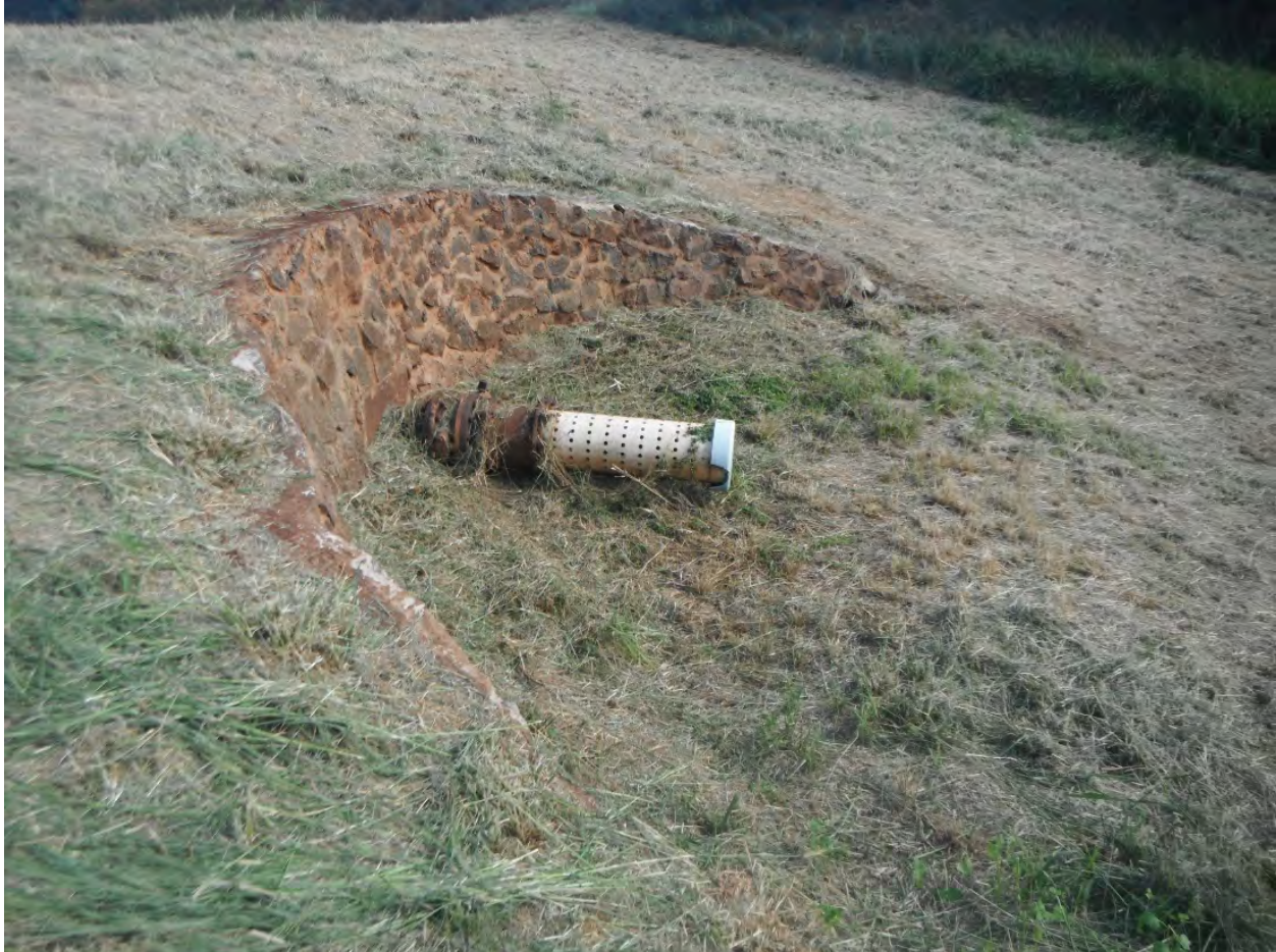
Figure 3- 9 Intake for the outlet pipe, Mahinahina Dam
